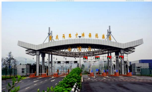
重庆保税港区水港功能区2.43 km 2 Water Port Section of CFTA
